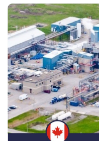
Welland, Canada Center for Solvay's phosphines platform
